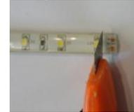
After cutting the flexible LED tape at the required size, remove silicone at the soldered joint.
